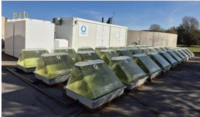
The Greek demo site evaluates the RHE-MEDIATION photobioreactor system under real operational conditions of a wastewater treatment plant. It is located at the Thriasio WWTP, operated by EYDAP, which services surrounding municipalities and local industries, discharging into the Gulf of Elefsis.
